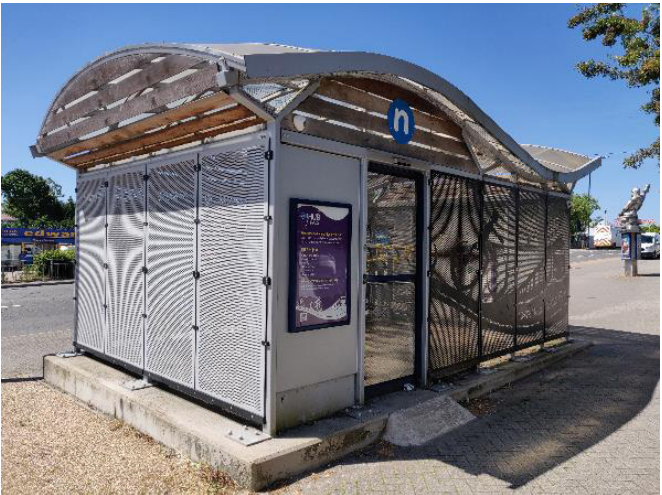
Figure 4.1: Use of mesh and clear polycarbonate panels and prominent location outside station adds to security of this unstaffed secure cycle parking hub.
