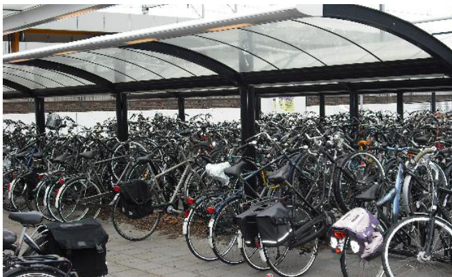
Figure 5.1: These high-low stands are popular in the Netherlands to maximise use of the space. The design doesn't work well for the UK due to the diversity of cycles in use and the fact that only the front wheel can be locked to the stand.
