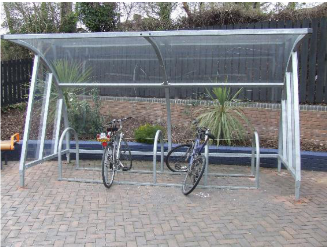
Figure 6.4: Toast rack parking in shelter at highly visible location. Good spacing between stands but the upstand of the horizontal metal bars at ground level results in the front wheel turning and some bikes may fall over. A flatter profile section can prevent this.
