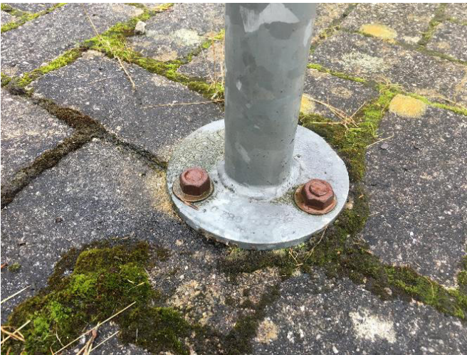
Figure 6.3: Insecure fixing with standard nut and bolt set in block paving.
